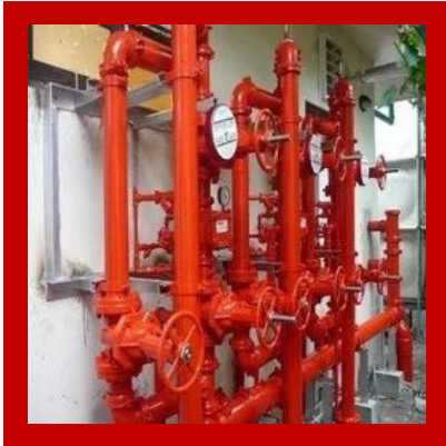
Fire Hydrant System Installation Services
