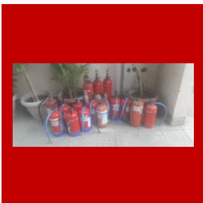
Fire Extinguisher Refilling Service
